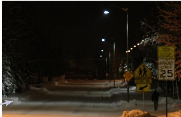
This test street in Anchorage, Alaska, USA compares the quality of light from warm, low CCT\* LEDs (right foreground), high pressure sodium vapor (left middle) and cool, high CCT LEDs (right background). The residents of this street preferred the warm LEDs in the foreground.
